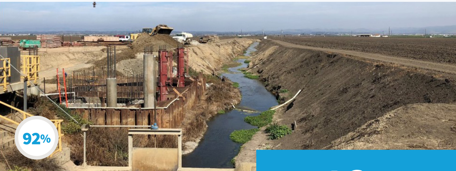
Source Water Diversion Structures
