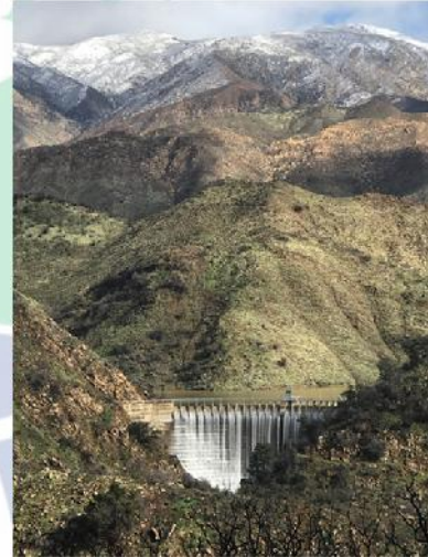
Water Education Foundation August 28, 2019
